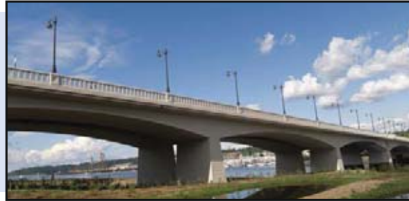
Concrete Box Girder
